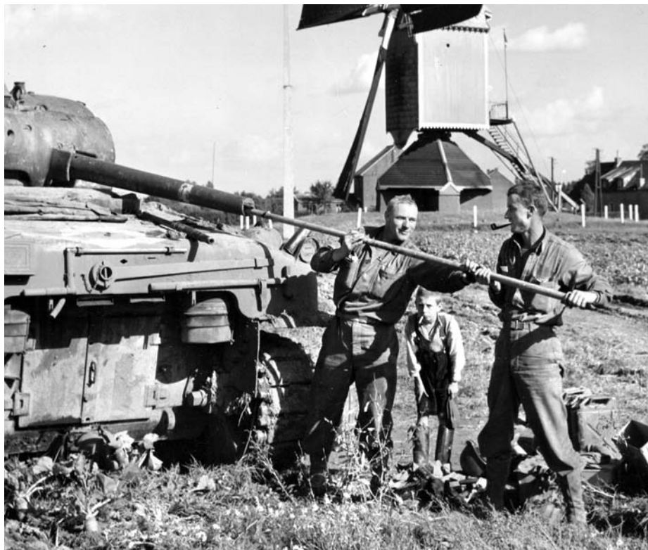
ABOVE: Near a windmill at Hasselt, Belgium, a young boy watches as tank crewmen clean the bore of their gun, September 1944. Crews often performed their own maintenance for simple jobs, leaving the difficult ones for the trained ordnance personnel. OPPOSITE: A 3rd Armored Division Sherman (right) passes a knocked-out Pz.Kpfw V "Panther" tank on a snowy Belgian forest road during the Battle of the Bulge, December 1944. A curious GI can be seen examining the enemy tank.
