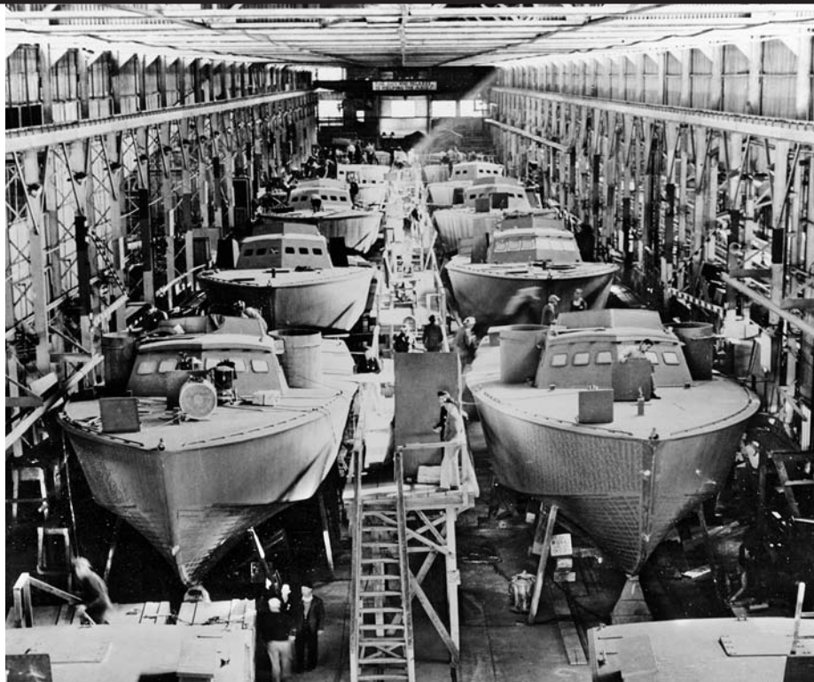
ABOVE: PT boats under construction on the assembly line at the Higgins Industries City Park Plant in New Orleans, Louisiana, during World War II. Other manufacturers, such as Elco, also produced the swift craft; a total of 531 were built. OPPOSITE: Three PT boats— PT-281 , PT-277 , and PT-288 (left to right) of Motor Torpedo Boat Squadron 23—are commissioned at the Higgins Industrial Canal Plant on June 28, 1942. Higgins had 20,000 employees working at seven different plants during the war.
