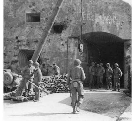
ABOVE: American soldiers mill around the entrance to Eben Emael in 1945. Damage from shell fire is apparent in both photos. TOP: The battle-scarred façade of the main entrance to Eben Emael has changed little since its capture by daring German paratroopers in 1940.
