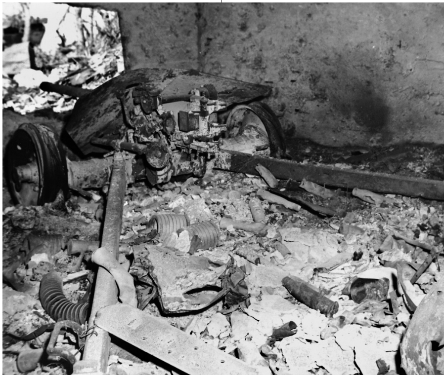
ABOVE: A destroyed Japanese 47mm antitank gun is shown in a photo taken well after the battle. It appears that the shell that knocked out the gun most probably entered through the embrasure. OPPOSITE: A view of the rear entrance of a camouflaged Japanese concrete antitank position. Note that the bunker was not scathed by the prelanding bombardment. It had to be taken by infantrymen with bayonet and rifle.
