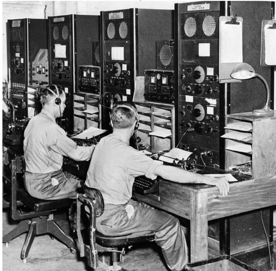
JCAA Radio Communications receiving positions at NAS, San Juan, Puerto Rico.
