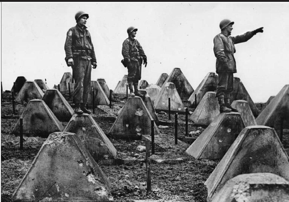
ABOVE: Members of a U.S. Army engineer unit stand on "dragon's teeth" antitank obstacles in a portion of the West Wall. RIGHT: An American soldier of the 4th Armored Division inspects one of three German panzers of the 11th Panzer Division knocked out during fighting near Guébling, France, about 30 miles southeast of Metz, on November 14, 1944.
