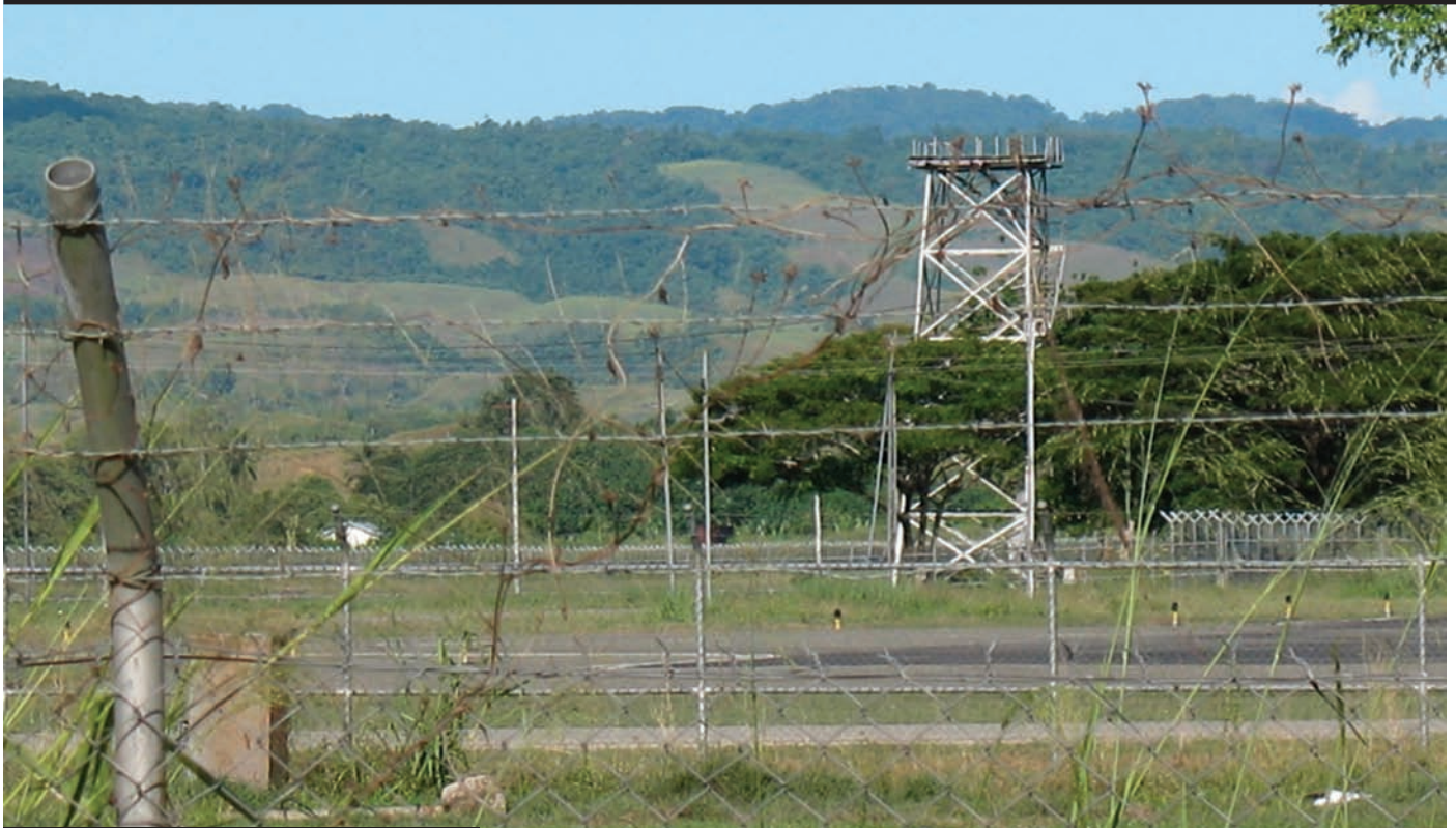
The skeleton of the Henderson Field control tower, built in 1943, sits on the edge of the runway of what is now known as Honiara International Airport.
