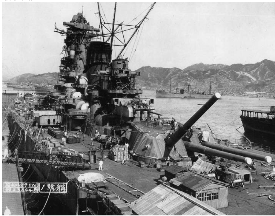
ABOVE: The Yamato is pictured on September 20, 1941, during the late stages of construction at the Kure Naval Base. Her armament included nine 18-inch main guns that could fire 3,200-pound shells a maximum range of 25 miles. BELOW: An illustration of the Yamato as she appeared at the time she was sunk.
