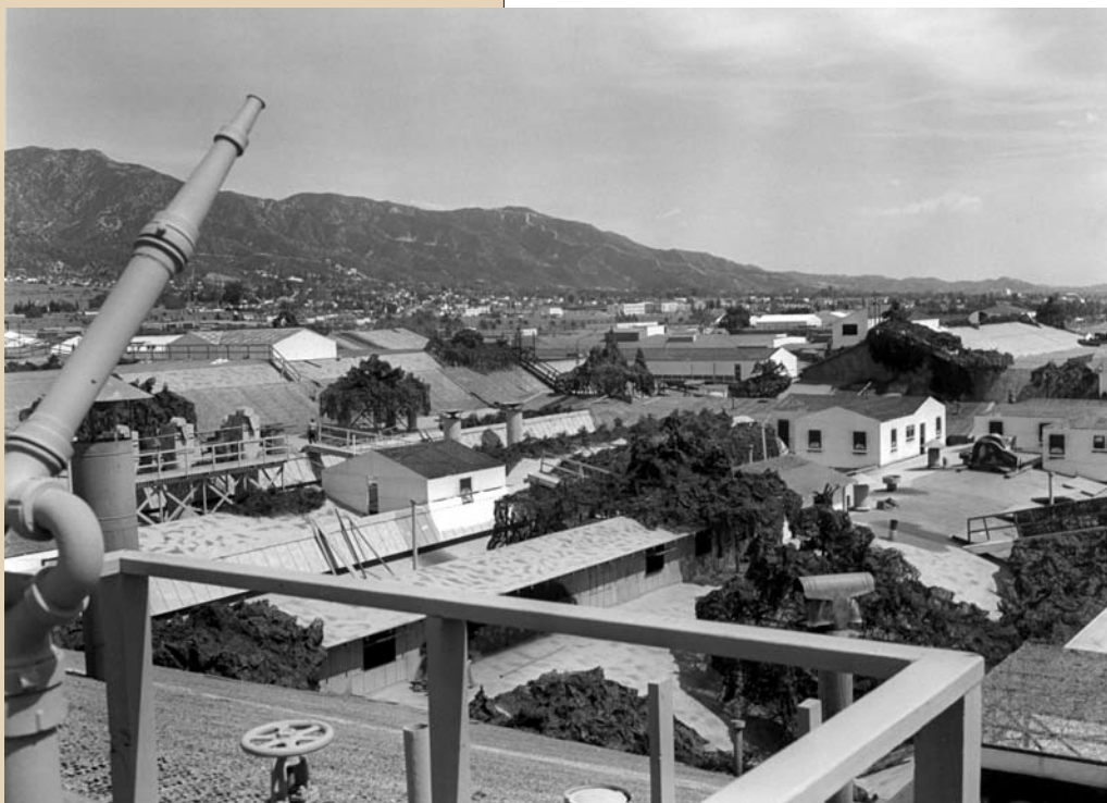
In this view of the Lockheed factory camouflage at Burbank, looking southeasterly toward Glendale, one gets an idea how complex much of the structure really was. On the left in the foreground is a hose nozzle for firefighting. Being made of wood, burlap, and tar, the whole affair was a potential fire hazard.
