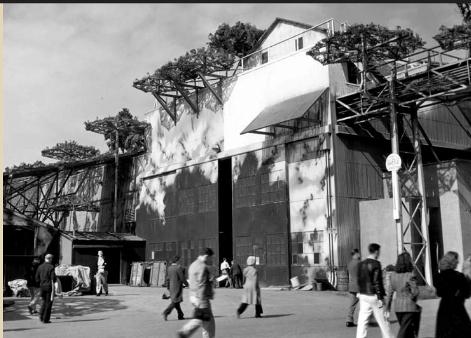
In areas at Douglas in Santa Monica where the camouflage netting ended with buildings, the edges were "softened" through the addition of artificial trees mounted on brackets.
