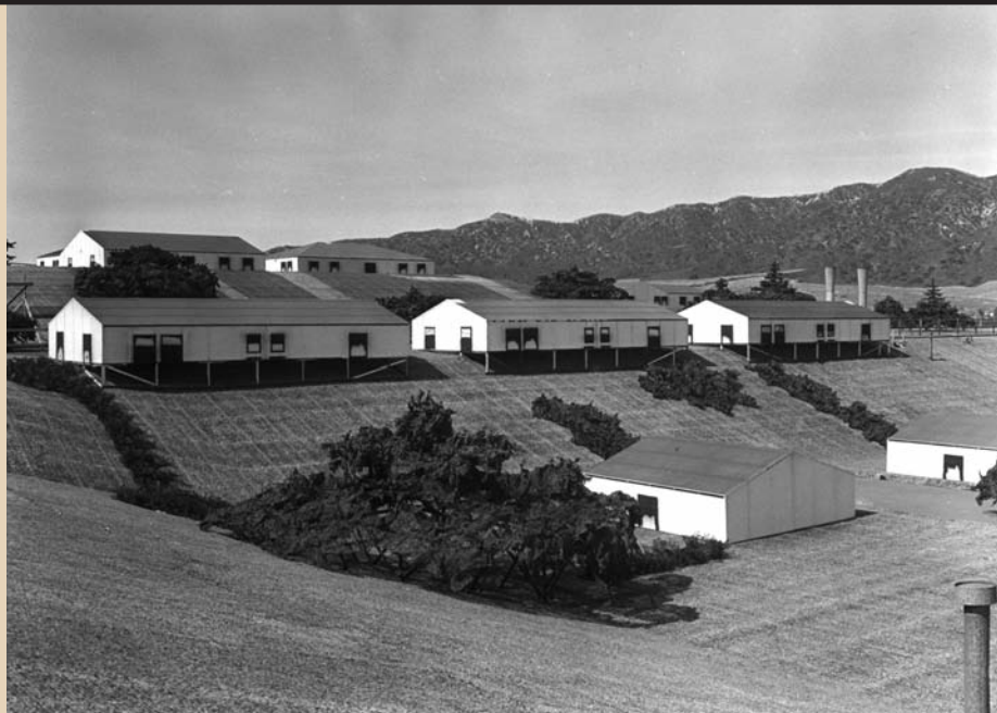
The rolling burlap hills of the subdivision top the rounded Lockheed factory roof in Burbank, with the San Gabriel Mountains in the distance.
