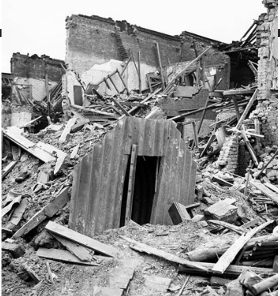
ABOVE: An Anderson bomb shelter remains largely intact and the three people inside were not harmed despite the devastation surrounding it when a German bomb landed nearby on Latham Street. OPPOSITE: On April 26, 1945, four years after the Blitz had ended, a German V2 rocket struck 800-year-old Smithfield Market, causing heavy damage and 100 deaths.
