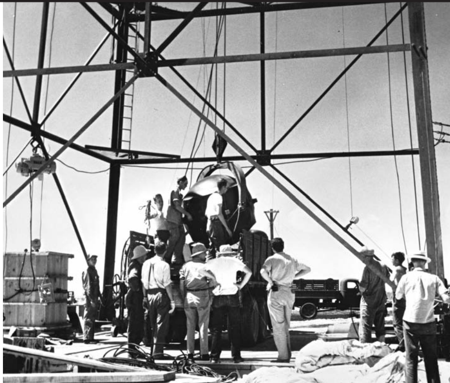
ABOVE: The Trinity test bomb, known as the “gadget,” is carefully winched to the top of a 100-foot tower for the final assembly at the Alamogordo Bombing and Gunnery Range, New Mexico. OPPOSITE: Alpha Track Calutron at the Y-12 plant at Oak Ridge, Tennessee, was used to enrich uranium for the Manhattan Project. RIGHT: Close-up of the “gadget,” photographed in the shed at the top of the tower prior to the test firing.
