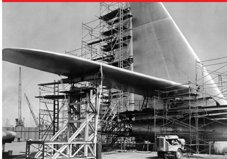
ABOVE: An aerial view of the H-4 Hercules shows its impressive size. The plane was almost 219 feet long from nose to tail and had a wingspan of 320 feet. BELOW: The tail of the H-4 was 85 feet—over five stories—high. The tail was deemed unstable after the initial flight according to some accounts.
