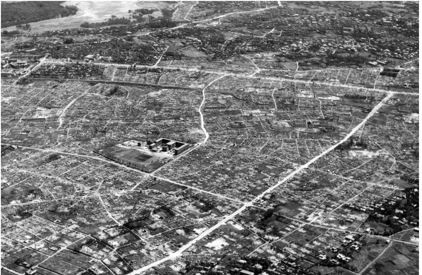
Looking more like Hiroshima after the atomic bombing, Tokyo, the world's third largest city, was reduced to rubble by war's end.
