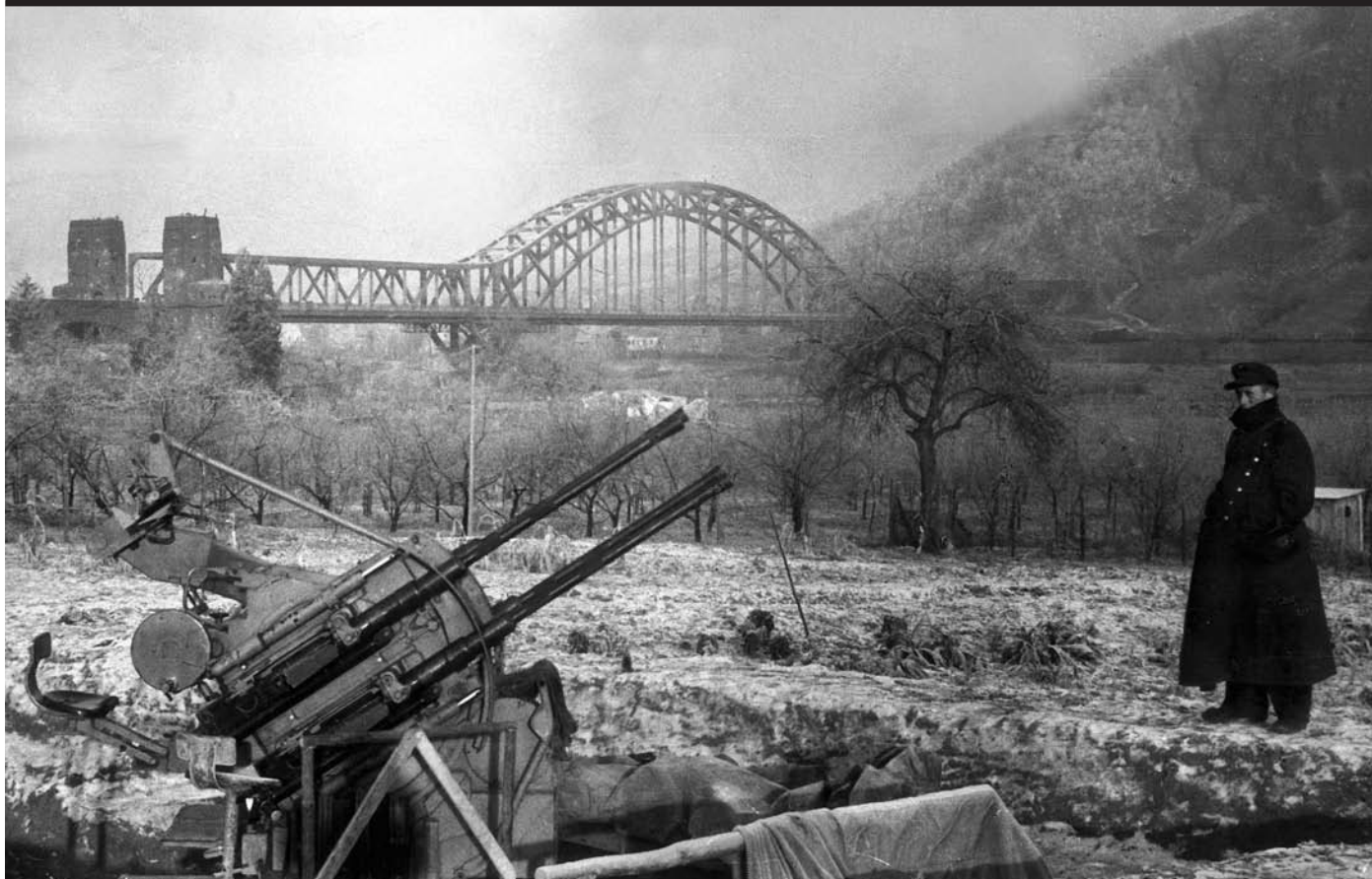
Bundled against the cold of late winter, a German soldier contemplates a 20mm anti-aircraft gun emplacement on the banks of the Rhine River. The Ludendorff Railroad Bridge with its great arch looms in the background. This photo was taken in January 1945, two months before American troops and tanks of the 9th Armored Division captured the bridge.
