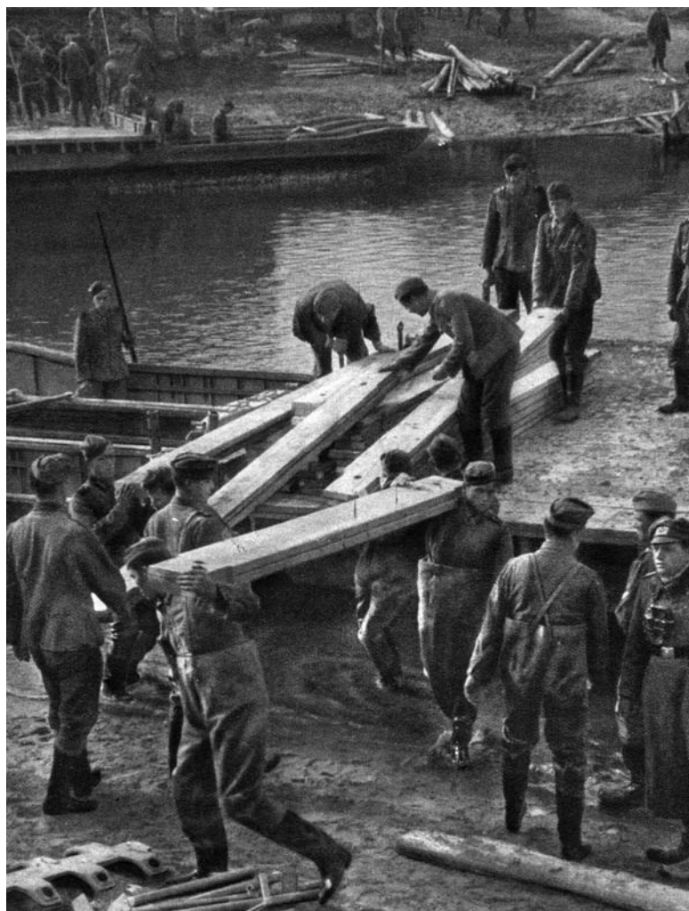
German pioneers (combat engineers) build a bridge over the Dnieper River to replace one that was destroyed by the retreating Red Army.
