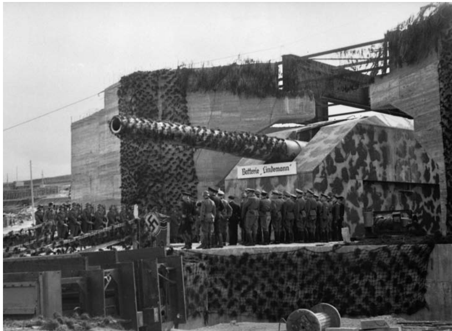
Although the steel-reinforced concrete roof has yet to be poured, Batterie Lindemann, with its 406mm Krupp naval gun, is commissioned in 1942.
