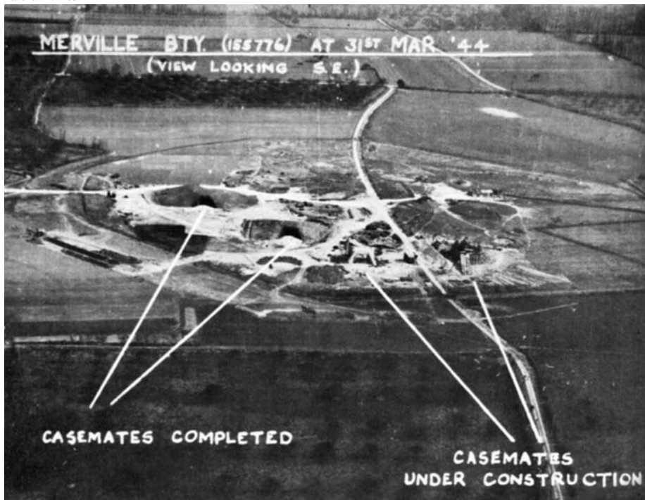
In an oblique shot of the Merville Battery taken by the Photo Reconnaissance Unit of the RAF, construction is underway on Casemates 3 and 4, while 1 and 2 are completed.
