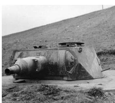
Large cement mixers pour the concrete for one of the casemates at Batterie Todt, the largest battery in France, located near Calais. RIGHT: A tank turret on Omaha Beach. The Germans frequently incorporated the turrets of captured enemy tanks into their fortifications.
