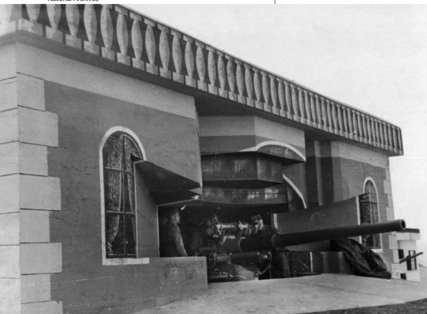
A Type 671 casemate at St.-Jean-de-Luz cleverly disguised to look, at least from a distance, like a house.
