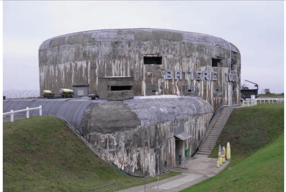
ABOVE: Turm I of Batterie Todt today. The “windows” of the bunker-turned-museum were used to vent the buildup of gases inside the casemate when the 38cm gun was fired. OPPOSITE: An enormous 406mm gun points menacingly toward the English Channel from one of the casemates at Batterie Lindemann. The thick concrete walls and roof were impervious to shellfire; the casemates could only be taken out by infantry assault.
