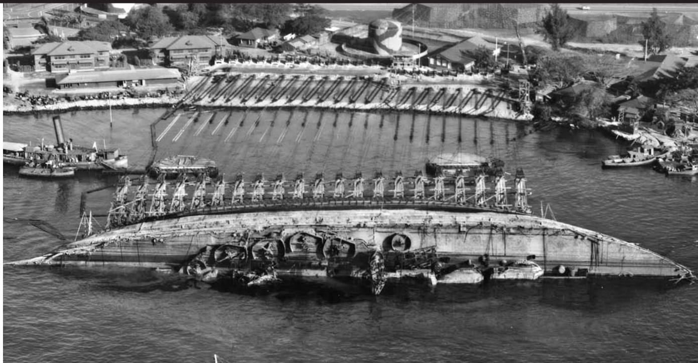
Winches from Ford Island attached to Oklahoma are used to right the ship, a process that took three months. The Japanese did not believe that the sunken ships could be salvaged to fight another day.
