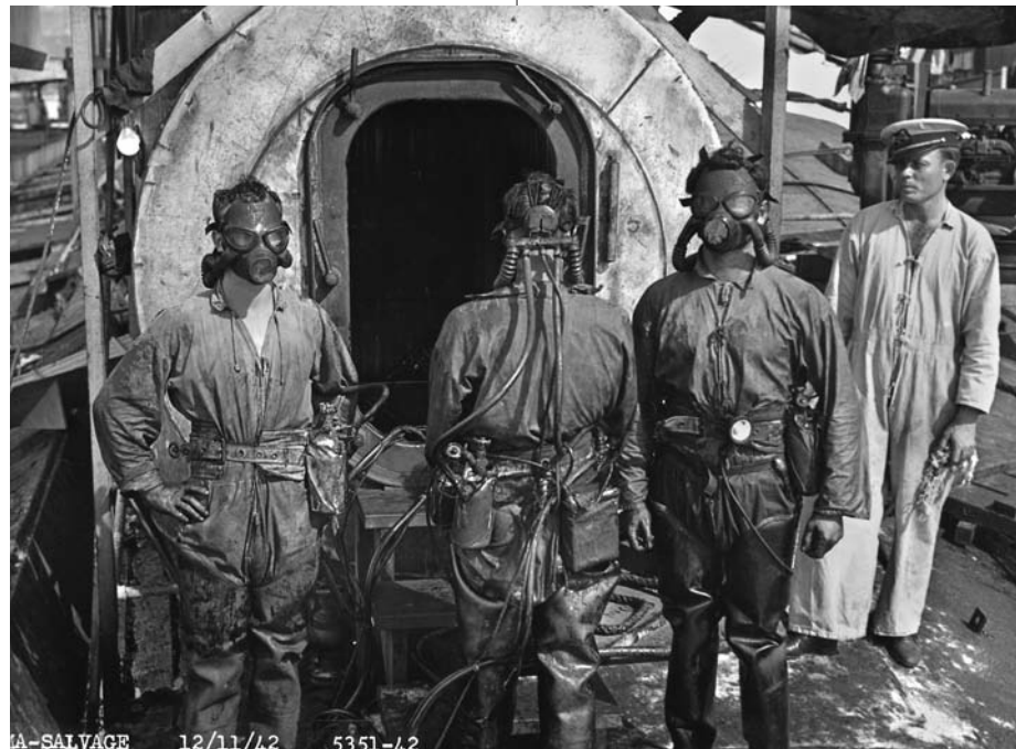
Navy salvage personnel equipped with face masks, air supply, and battery-powered miner's lights come off their shift aboard Oklahoma , December 1942. While initial plans were made to salvage the ship, the Oklahoma was decommissioned in 1944.
