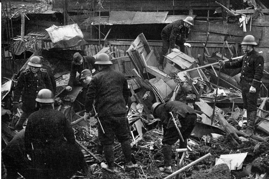
ABOVE: Firemen and Civil Guards attempt to find victims in the wreckage of a Tokyo building. BELOW: The 1,800-degree heat generated by the March 9/10 firestorm instantly cremated residents of Tokyo. It is estimated that 90,000-100,000 Japanese died during Operation Meetinghouse. OPPOSITE: The devastation caused by the fire-bombing was widespread over much of Tokyo. Only brick and concrete buildings stood a chance of survival. Despite the damage, the Japanese government refused to surrender—until two atomic bombs were dropped on Hiroshima and Nagasaki in August 1945.
