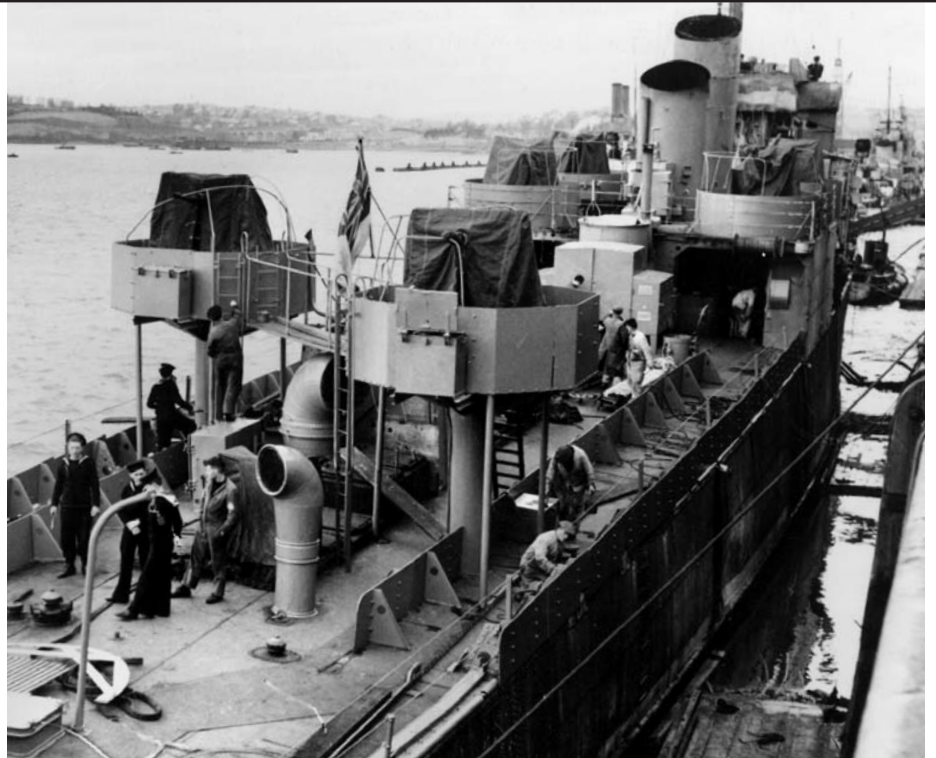
A view of HMS Campbelltown (formerly the USS Buchanan ) shortly before leaving Devonport for the raid. The ship has been modified to look like a German Möwe -class torpedo boat in order to fool the enemy. Besides carrying scores of Commandos, the ship was packed with 9,600 pounds of explosives and delayed-action fuses.
