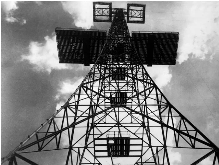
ABOVE: One of the many Chain Home Radar towers that stood guard along England's southern coast. Radar was then known as "Radio Direction Finding"—an early warning system that was simple but effective in detecting the approach of Luftwaffe formations over the English Channel. OPPOSITE: Flying wingtip-to-wingtip, a formation of RAF Hawker Hurricanes from No. 111 Squadron glides above the English countryside. While the Spitfire is more famous today, the Hurricane was the first monoplane fighter to exceed 300 miles per hour and accounted for many "kills" against the Luftwaffe.
