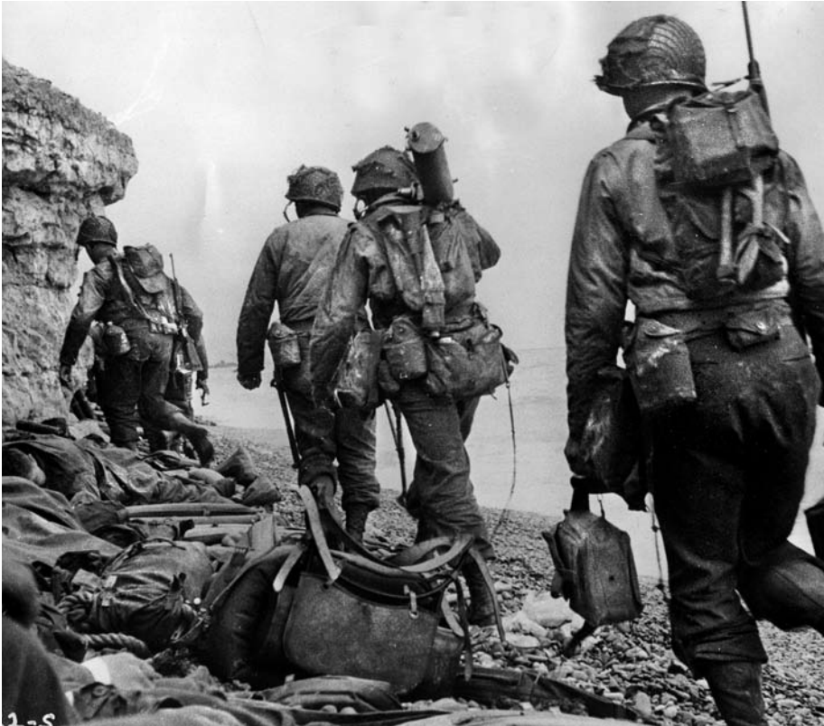
ABOVE: As the tide rises, the beach becomes narrower. Here a heavy machine-gun team makes its way toward to its assigned position along the equipment-littered shingle. OPPOSITE: A soldier's smoke grenade, apparently struck by a German bullet, explodes inside an LCVP, as the boat driver makes haste for the shore.
