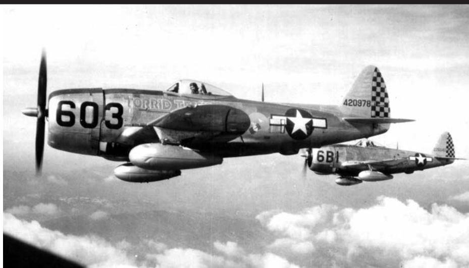
Two P-47D Thunderbolt fighters off the wing of a B-17. With their limited range, the P-47s could not accompany the bombers to distant targets, but P-51s could.
