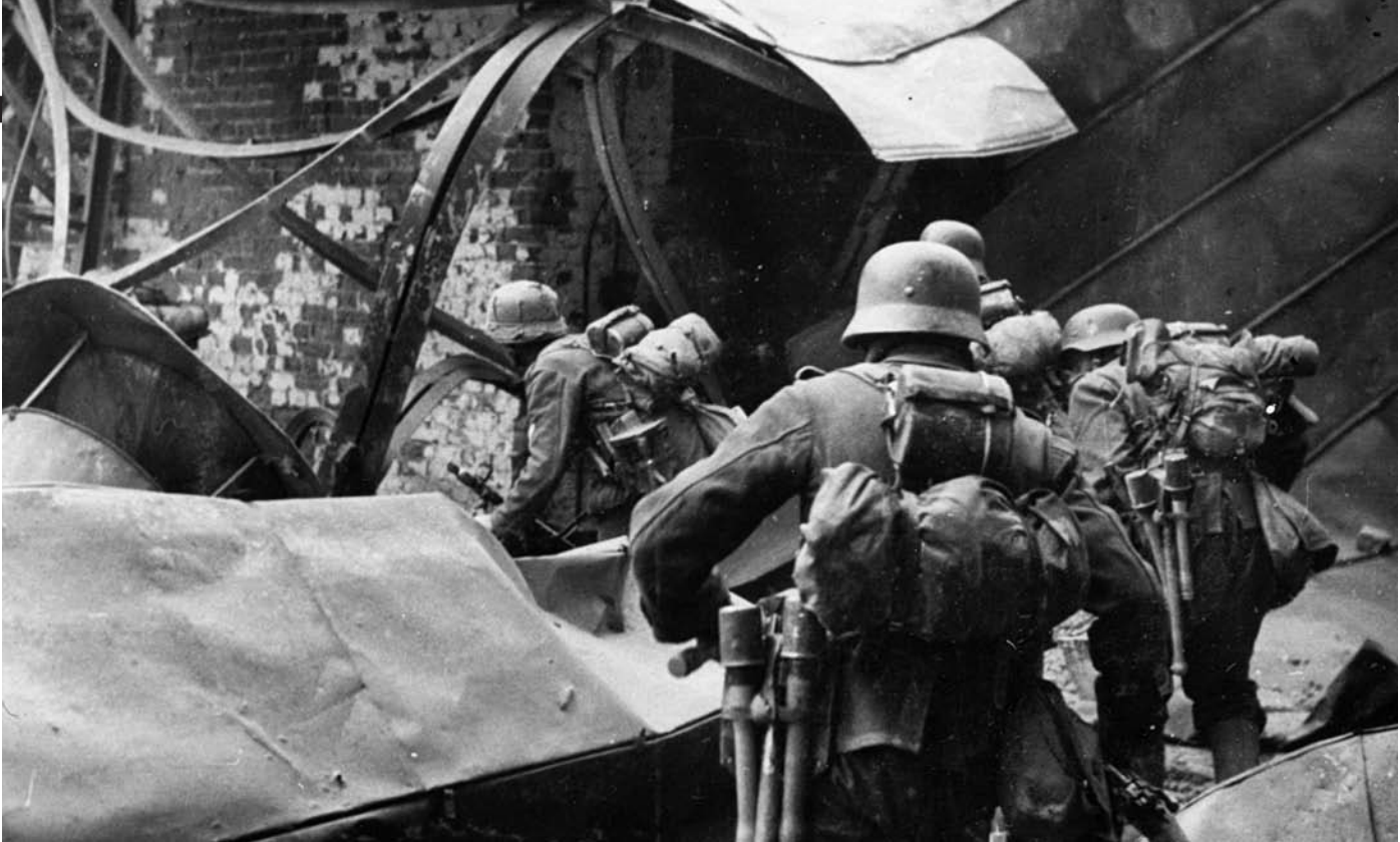
ABOVE: German troops enter the ruins of the "Red October" factory, autumn 1942. The Soviet troops used the extensive rubble of Stalingrad as cover, emerging from their hiding places to inflict heavy losses on the Wehrmacht. OPPOSITE: Leaving its target along the Volga River on the outskirts of Stalingrad burning, a Stuka dive bomber pulls up and heads for its home base.
