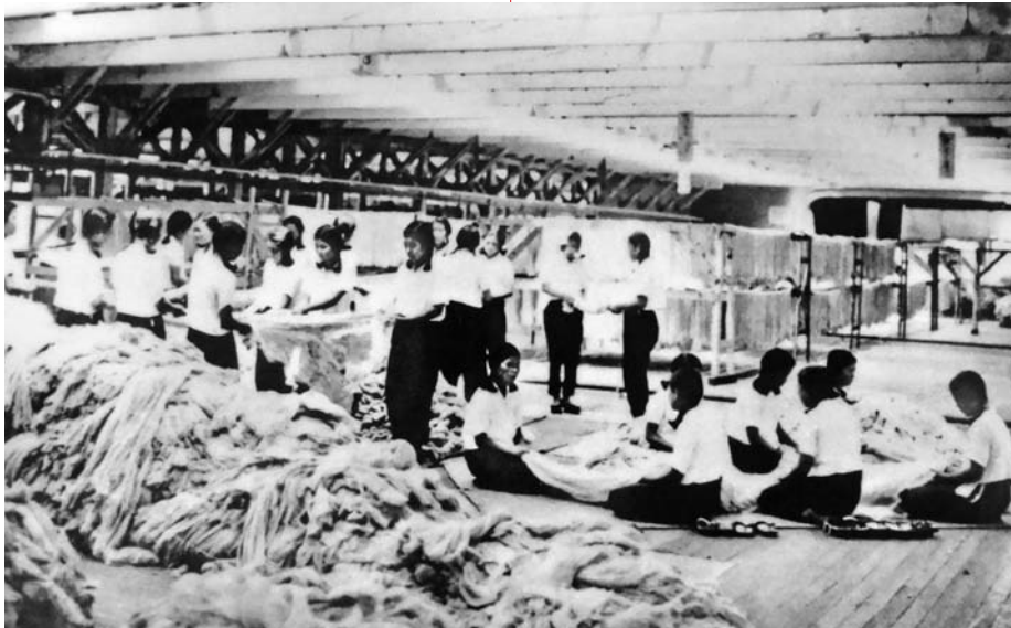
ABOVE: Due to Japan's shortage of rubber, Japanese schoolgirls assemble sheets of paper made from the kozo bush that were used to construct the balloons. BELOW: Japanese schoolgirls push one of the giant balloons across a factory floor during final inspection.
