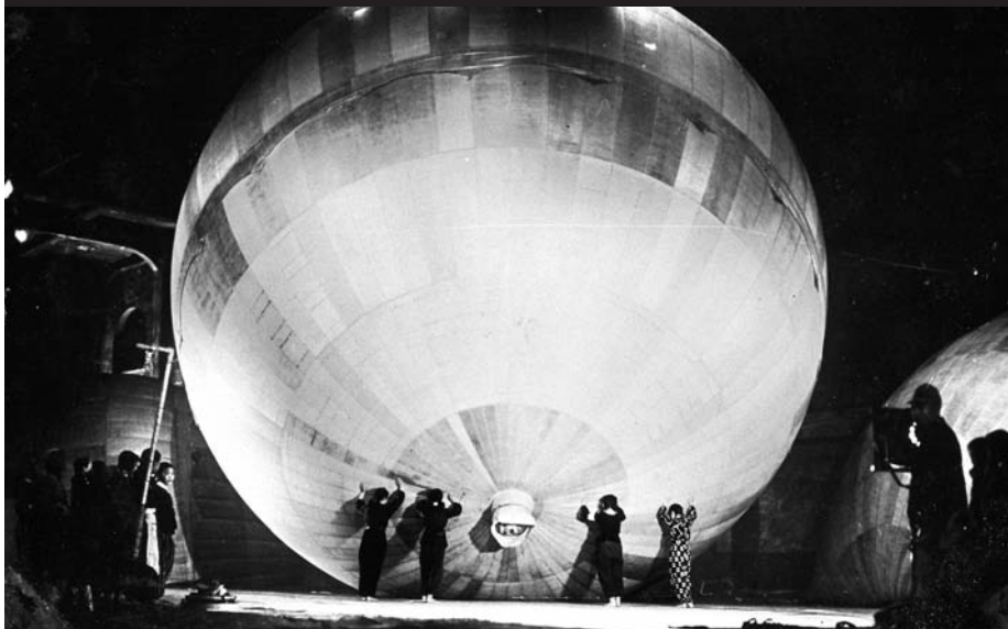
ABOVE: Due to Japan's shortage of rubber, Japanese schoolgirls assemble sheets of paper made from the kozo bush that were used to construct the balloons. BELOW: Japanese schoolgirls push one of the giant balloons across a factory floor during final inspection.
