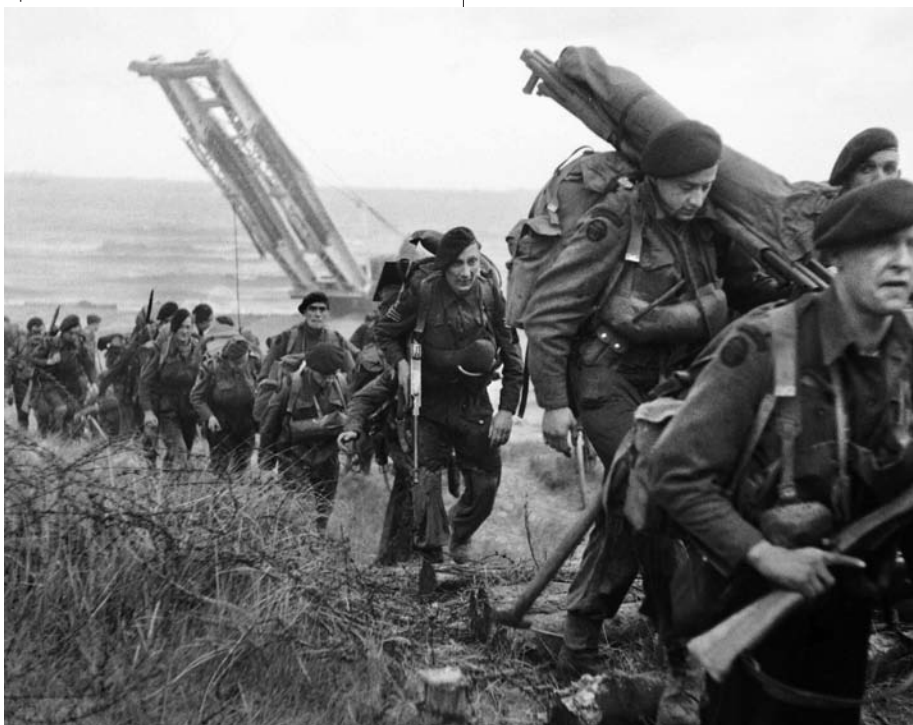
Royal Marine Commandos of 1st Special Service Brigade move inland from Queen Red beach. A Churchill AVRE tank with raised girder bridge is visible in the background.
