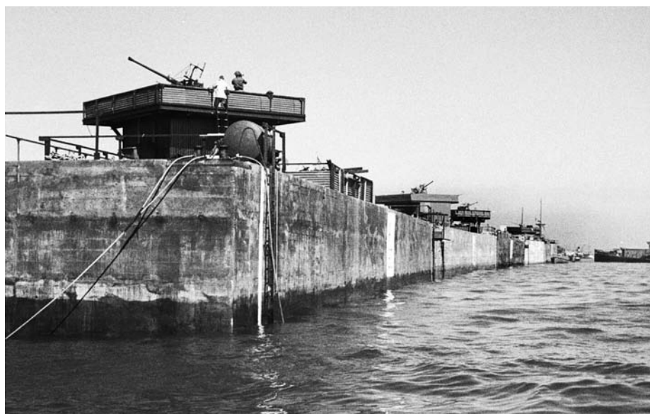
ABOVE: Seacocks were opened to allow water to sink them into position. Antiaircraft guns were mounted on the largest caissons and barrage balloons floated overhead as protection against enemy aircraft. TOP: Caissons were moved into position by tugs to form a continuous line of breakwaters. OPPOSITE: Aerial view of the Gooseberry breakwater that was emplaced hours after the Normandy landings at Arromanches. Vessels can be seen passing through openings in the line of old Navy ships sunk to create the Gooseberry.
