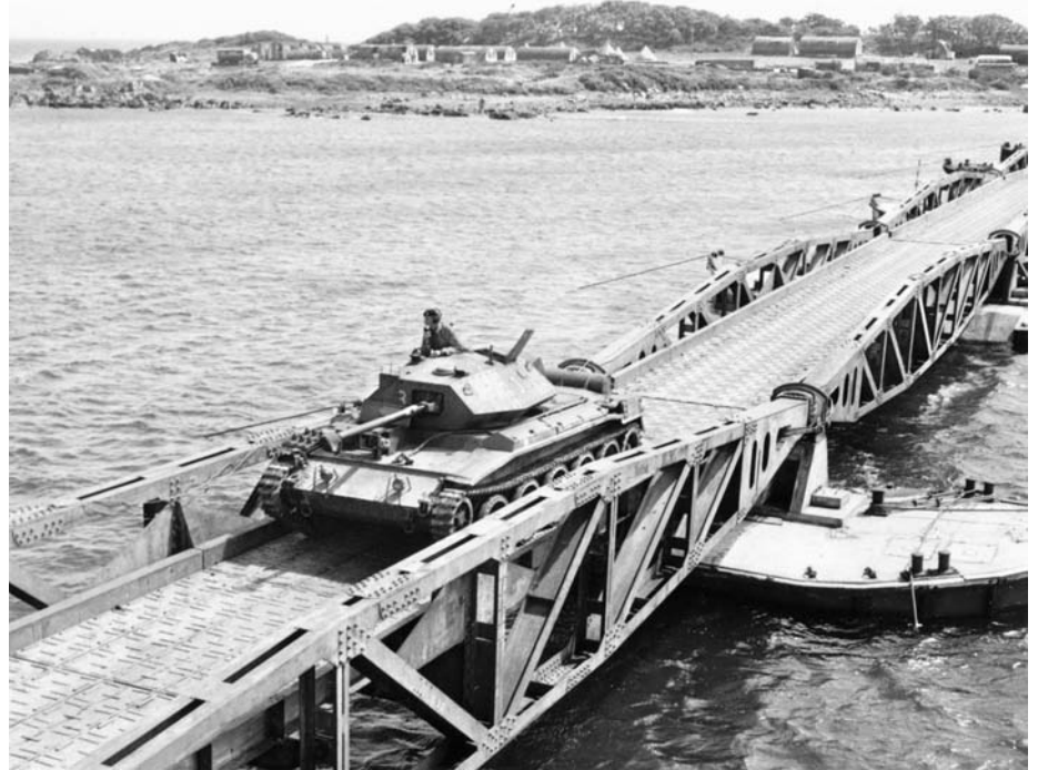
ABOVE: As testing nears completion, a British Crusader tank heads away from Cairn Head in Garlieston Harbour, Scotland, on Allan Beckett's floating roadway. This location was selected because the tide there rises up to 24 feet, similar to Normandy. OPPOSITE: Dwight Shepler painted the massive concrete "Phoenix" caisson units under construction at Portsmouth, England. These were then towed across the English Channel at 3-4 knots, where they were then sunk to create the breakwaters.
