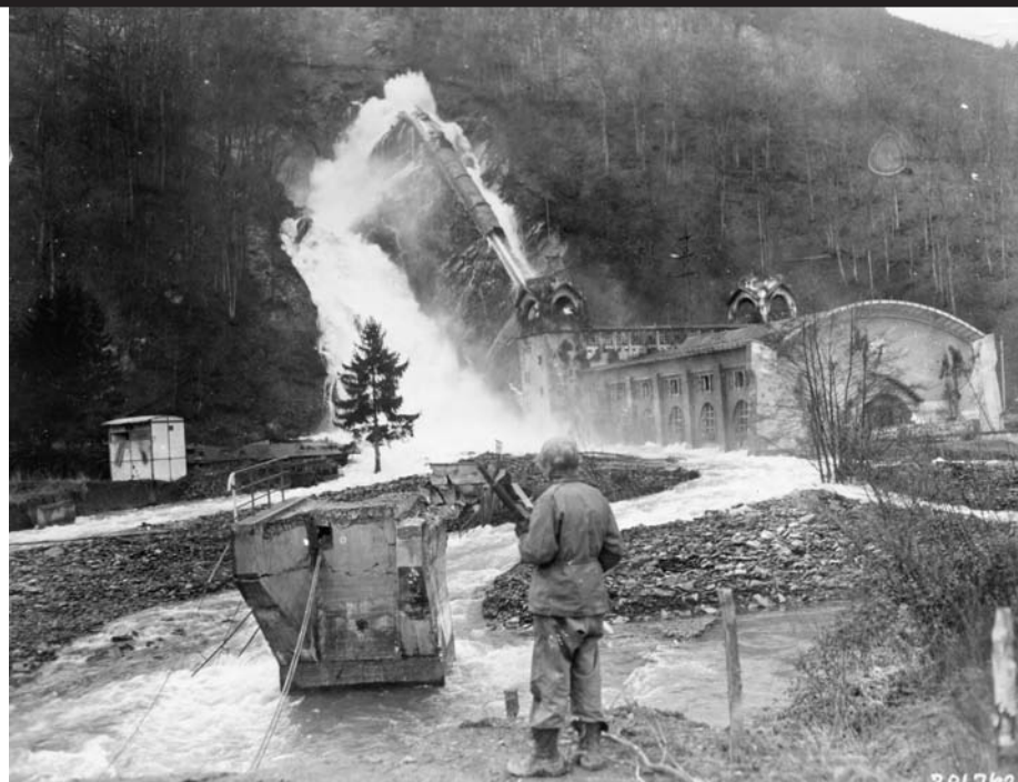
ABOVE: An American soldier watches torrents of water from the River Rur flow around the Heimbach hydro electric plant after the Schwammenauel Dam was breached in February 1945. OPPOSITE: A line of American troops crosses a bridge and marches through one of the many small villages that dot the Hürtgen region. The difficult hilly and forested terrain is very obvious in this photo, taken November 16, 1944.
