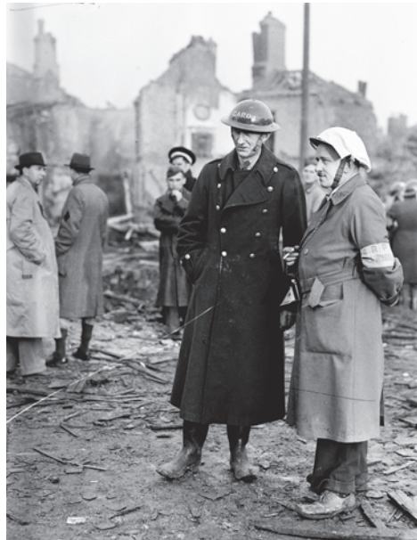
ABOVE: Two Dublin officials view damage in the North Strand, Dublin, May 31, 1941, and perhaps search for answers as to "why." OPPOSITE: Extensive wreckage in the North Strand, Dublin, after the May 31, 1941, raid that killed 34 civilians, wounded 90, and destroyed or damaged nearly 70 homes.
