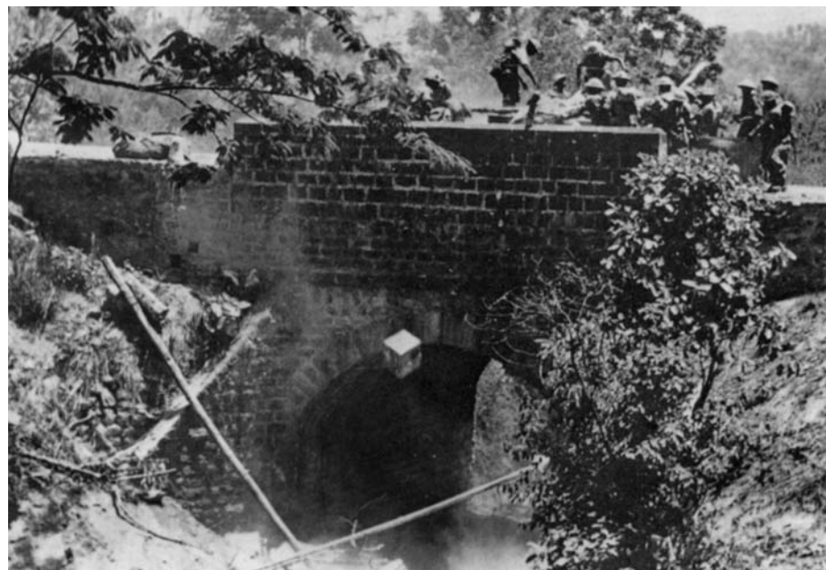
ABOVE: Sappers clear obstructions from a barricaded bridge. The Japanese moved through back country to descend on roads and set up their blockades. OPPOSITE: Two men stand beside trenches of DIS Ridge near Kohima. In the distance is Naga Village. Intense fighting took place along this line.
