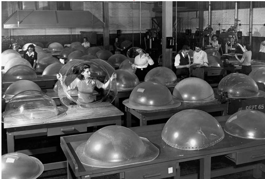
Employees inspect plexiglass “blister” dome windows. The B-29 was produced at four factories around the United States.
