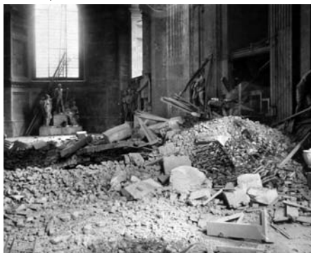
ABOVE: St. Paul's did suffer some damage, including this caused by falling debris. On the whole, however, the structure survived with minimal damage; many believed that the cathedral was saved by divine intervention. BELOW: Much of central London was a smoldering, burned-out hulk. This view, taken the day after the raid, shows Ludgate Circus with St. Paul's in the background.
