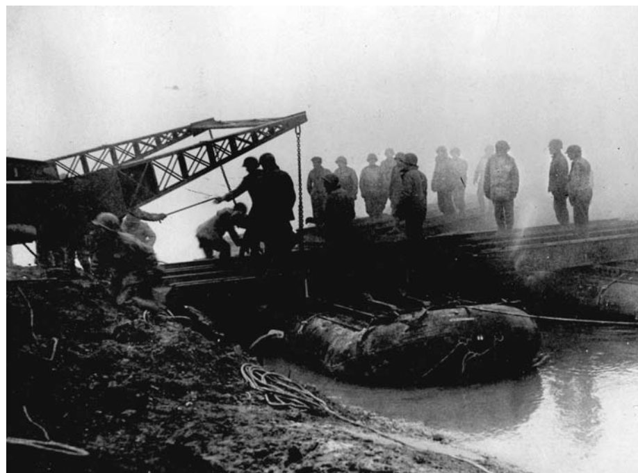
Third Army engineers complete installing the first section of a pontoon bridge across the Moselle River, allowing for the resupply of American forces assaulting German-held Metz.
