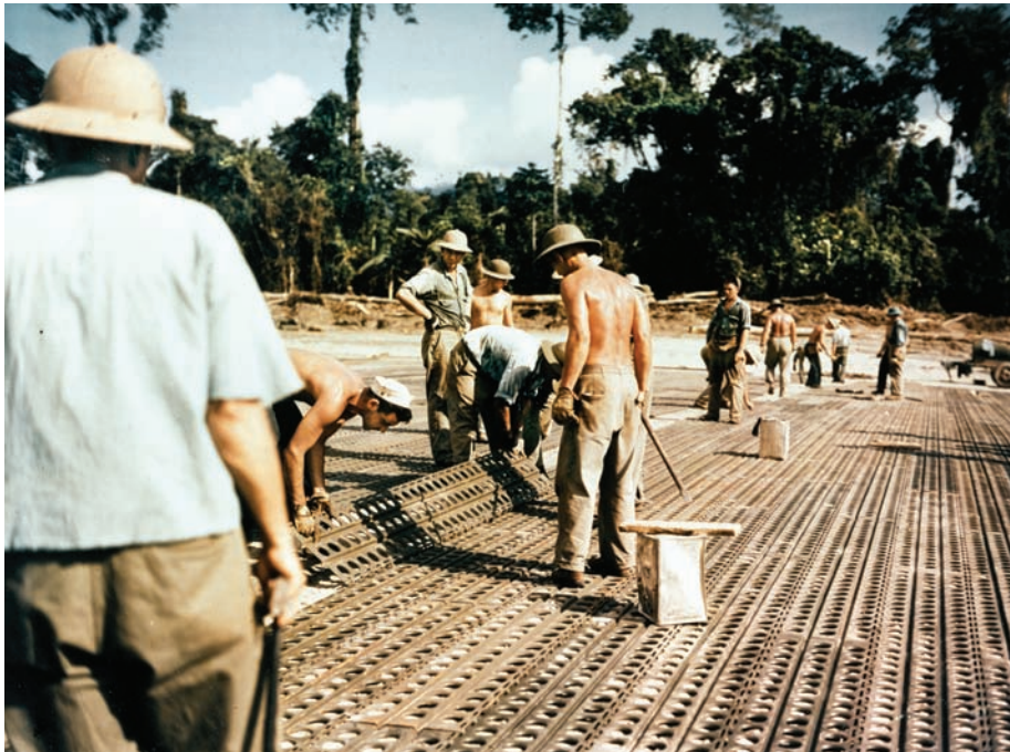
ABOVE: Seabees lay steel mats during the construction of a new bomber airfield on Bougainville, December 1943. BELOW: The Torokina fighter airstrip on Bougainville, one of the main objectives of the March 1944 Japanese counterattack. Note the Allied shipping in Empress Augusta Bay.
