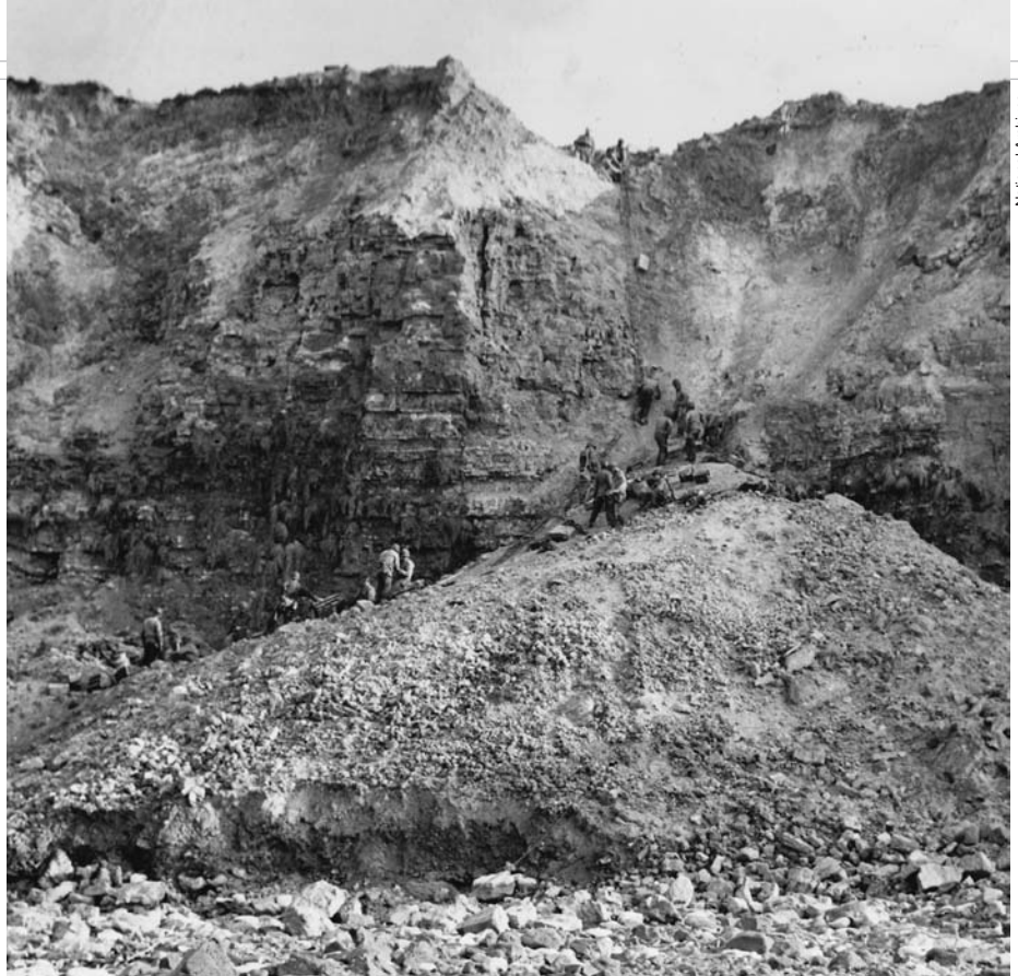
ABOVE: Using a mound of dirt and debris created by pre-invasion shelling and bombing raids, American troops raise supplies to the top of Pointe du Hoc. Only 99 of the attacking Rangers came through the bitter fighting on D-Day unscathed. OPPOSITE: Taken after the fighting at Pointe du Hoc was over, this photo is indicative of the arduous task that faced the U.S. Army Rangers who assailed the German position atop the craggy promontory on D-Day.
