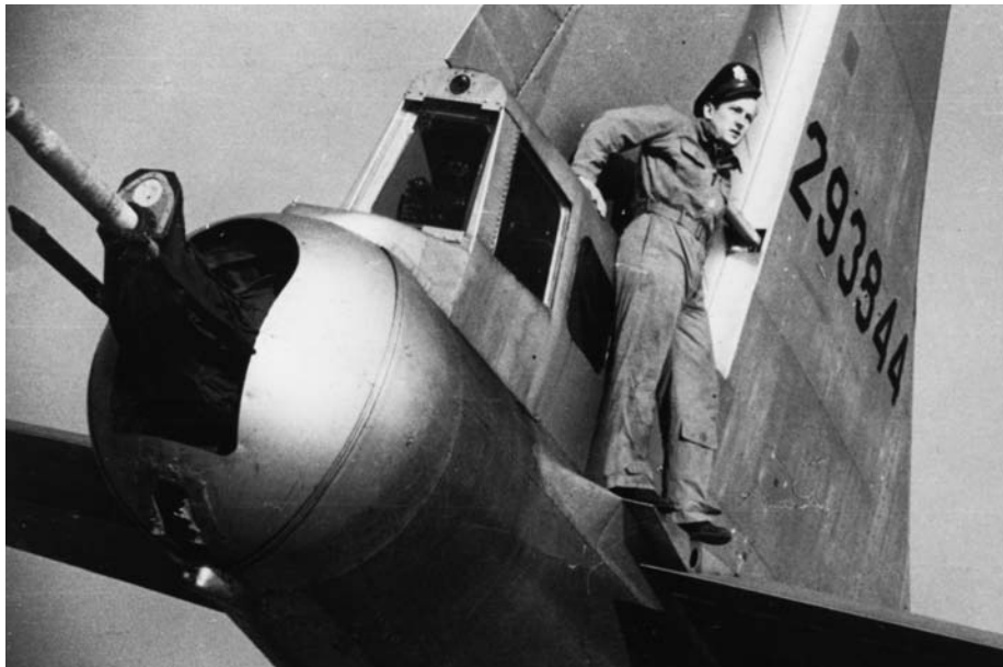
ABOVE: First Lieutenant George Wale stands on a B-29's horizontal stabilizer near the tail gunner's position. The centerline-mounted 20mm cannon and dual .50-caliber machine guns made the B-29 a formidable opponent for enemy fighters attacking from the rear. RIGHT: Recently graduated from gunnery school at Harlingen, Texas, in 1944, Andy Doty wears gunners wings on his uniform.
