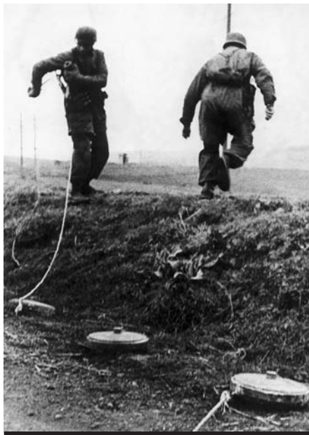
German airborne engineers place antitank mines on a dirt road in Italy near the towns of Anzio and Nettuno. Note that the mines are attached to cords so that they can be pulled from secure cover in the path of advancing Allied armor.
