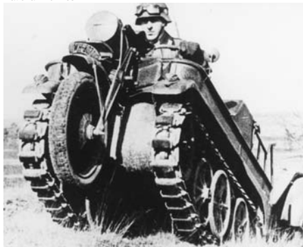
This famous photo was the first of the Kettenkrad to appear in wide circulation. It was originally published in the July 30, 1942, issue of The Illustrated Newspaper . The motorcycle steering and front assembly are readily visible, as is the large trailer following behind.
