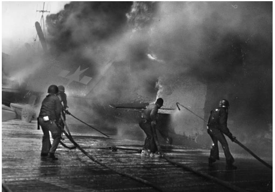
A damage control party works feverishly to extinguish fires aboard the USS Enterprise after the aircraft carrier was struck by a kamikaze and forced to withdraw from the fighting in the waters around embattled Okinawa.
