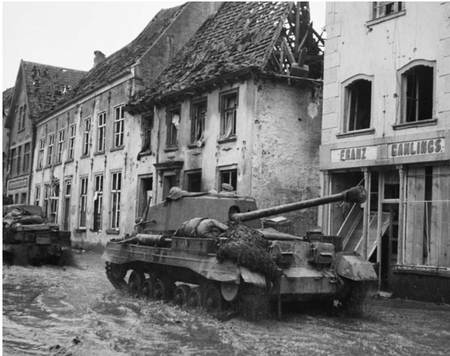
Photographed in the flooded streets of the German town of Kranenburg on February 11, 1945, these British Archer tank destroyers are attempting to reach the front. German defenders opened the gates of numerous dams and flooded extensive areas to slow British progress during Operation Veritable.
