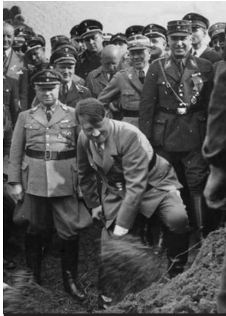
With Dr. Fritz Todt standing at right, Hitler turns the first spade of dirt to begin construction on the German Autobahn near Frankfurt in 1933.
