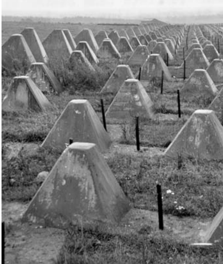
ABOVE: In this photograph snapped during the 1930s, a section of the modern Autobahn stretches into the distance across the German countryside. Note the service station at left. BELOW: Concrete antitank obstacles such as these studded the German West Wall, or Siegfried Line, along with wide ditches, fortified strong-points, and mines. The Siegfried Line was one of the many major construction projects supervised by Dr. Todt.
