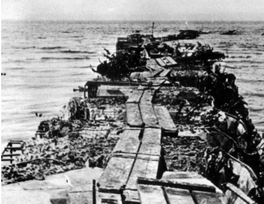
This makeshift jetty was constructed atop vehicles driven into the waters of the English Channel at Dunkirk allowing soldiers to board ships more quickly. BELOW: This iconic photo of British troops massed along the beach at Dunkirk provides a glimpse into the magnitude of Operation Dynamo. The sealift involved both military and civilian watercraft crossing the English Channel.
