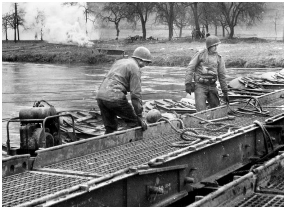
ABOVE: American combat engineers with the 5th Infantry Division erect a treadway bridge across the Sauer River. Smoke, intended to help protect the exposed engineers from enemy fire, billows after a shell has impacted the opposite bank. BELOW: An M4 Sherman tank of the 737th Tank Battalion has hit an icy patch and skidded off a road in Luxembourg while supporting the 5th Infantry Division’s movement toward German positions.
