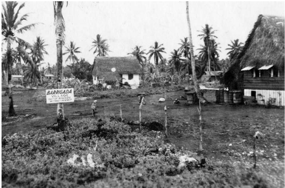
Soldiers of the 77th Division fought the Japanese for control of a precious water source at the village of Barrigada. The opposing forces clashed for two days, and both sides used tanks in the fight to take possession of the town's 30,000-gallon reservoir.
