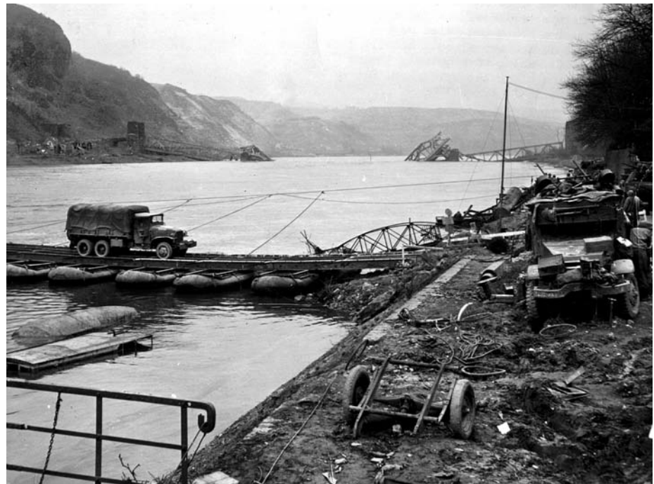
ABOVE: The remnants of the destroyed bridge are seen in the background of this photo depicting one of two pontoon bridges the Americans deployed to facilitate the movement of troops and equipment across the Rhine. OPPOSITE: The tunnel into the Epeler Ley cliff, where German soldiers and civilians took shelter during the fighting at Remagen, is visible at upper left in this photo taken in October 1945. The wreckage of the Ludendorff bridge, which had been heavily damaged during earlier fighting but miraculously remained intact for several days after its capture, lies in the foreground.
