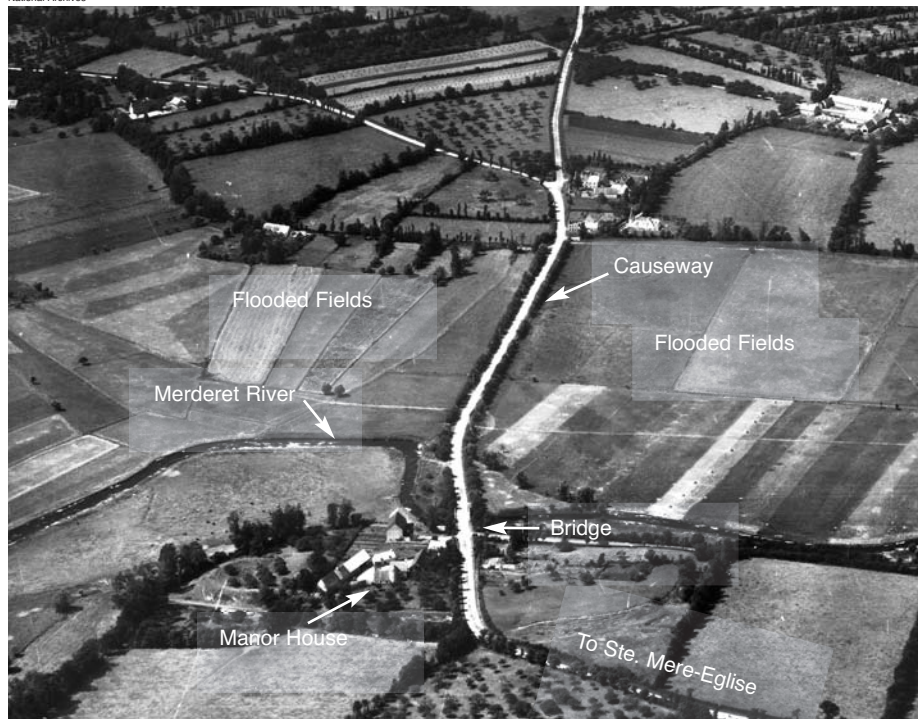
The La Fiere bridge is visible in the lower center portion of this aerial photograph, a few miles west of the town of Ste. Mere-Eglise. It stands just to the right of La Fiere Manor, the scene of fierce fighting during the early phase of the Normandy operation as American paratroopers retained control of the span. The large fields in the center of the photo were flooded by the Germans prior to D-Day, and they were virtually impassable in June 1944.
