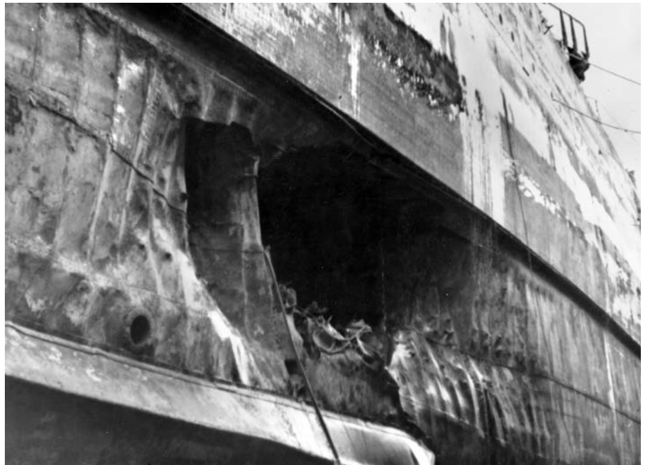
ABOVE: Torpedo damage to the hull of California , photographed at the Pearl Harbor Navy Yard in April 1942, after the ship had been dry-docked for repairs. Visible is the forward torpedo hole, showing the armor belt above the hole and bilge keel below it. BELOW: Painted in camouflage pattern Measure 32, Design 16-D, the repaired and modernized California steams at eight knots off the coast of Washington state on January 25, 1944. After returning to service, the battleship bombarded Japanese positions on several Pacific islands in support of amphibious landings.
