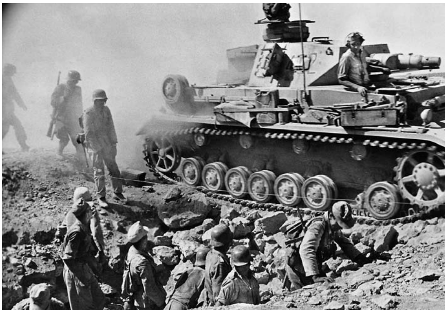
German engineers construct a bridge across one of the many tank traps that defended the approaches to Tobruk.
