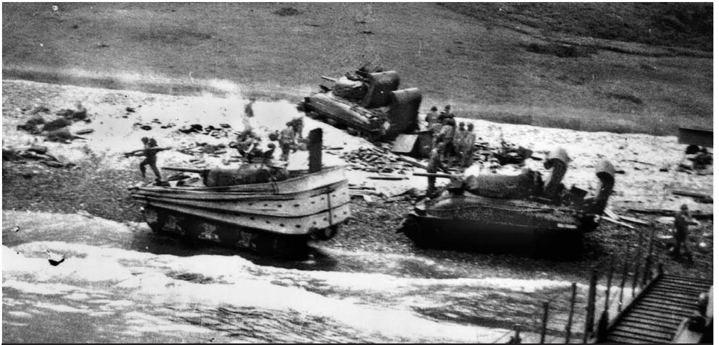
A duplex drive (DD) M4A1 Sherman medium tank on Omaha Beach on D-Day, June 6, 1944. Note that its canvas flotation screen is partially lowered. Also visible are two Sherman wading tanks, incorporating waterproof hulls and tall intake and exhaust vents that allowed them to operate in shallow water.
