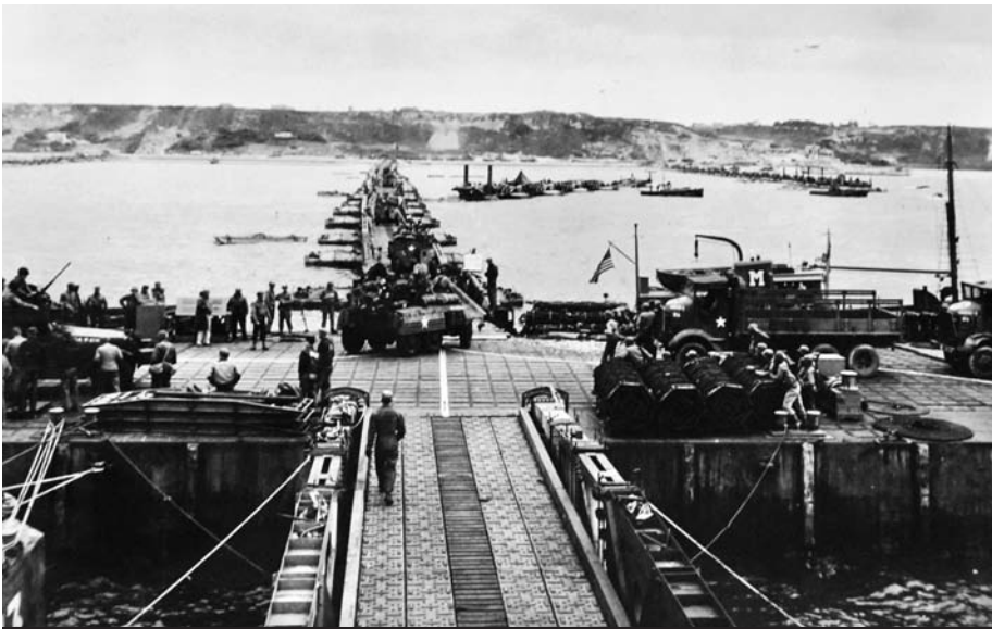
This view from the pier head of a Mulberry harbor shows the roadway to the invasion beach in Normandy. This vertically moving pier head maintained a fixed level above the changing surface of the sea.
