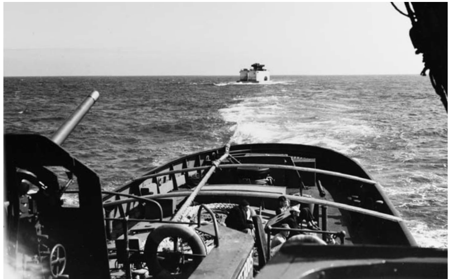
A Phoenix caisson is towed across the English Channel toward the beaches of Normandy. These components were towed at speeds of just three or four knots.
