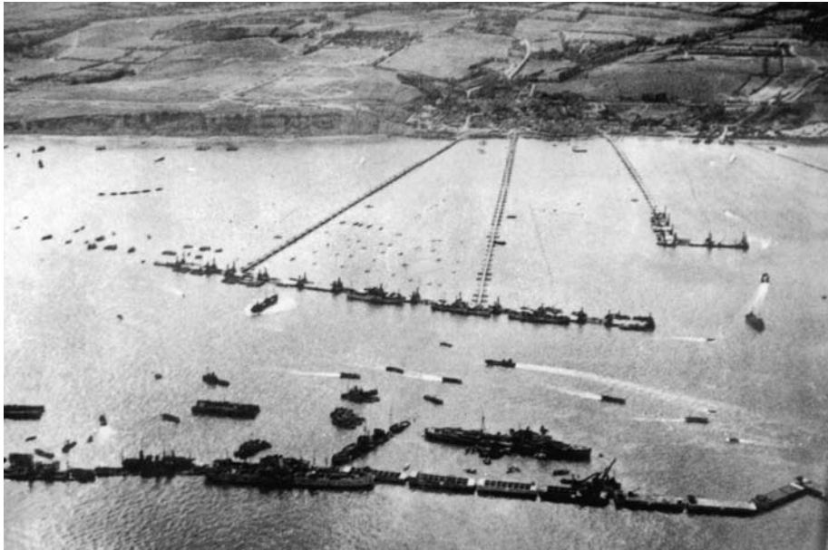
This aerial view depicts a Mulberry harbor completely deployed off the coast of Normandy and in full operation. The breakwater consisting of caissons and block ships is shown at bottom, while the row of pier heads forms a wharf at center, and the floating roadways run directly toward the beach. When fully assembled, a Mulberry harbor was roughly the same size as that of Dover, England.
