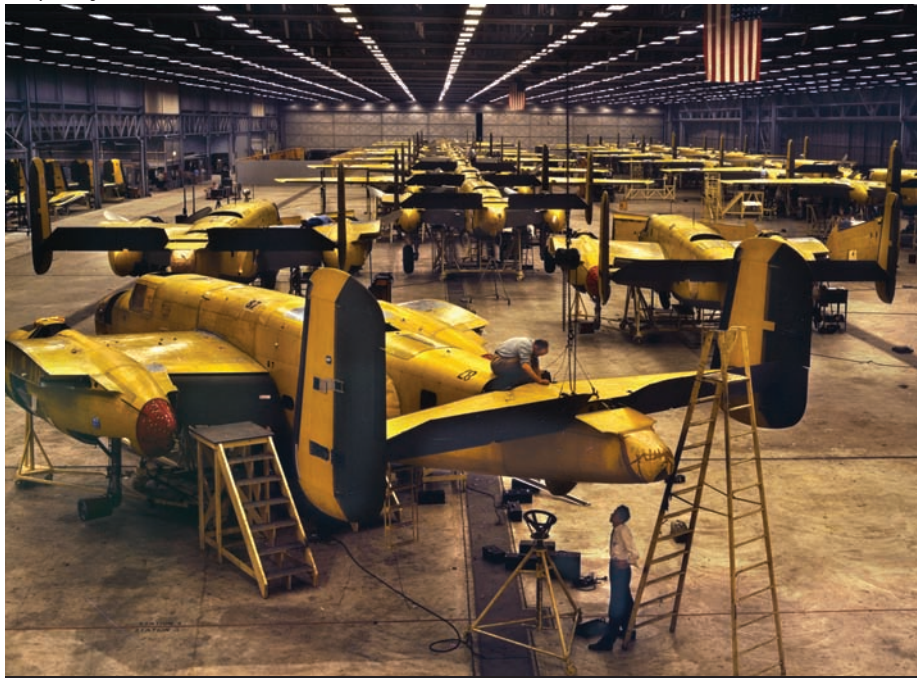
ABOVE: Workers assemble B-25 Mitchell medium bombers on the floor of the factory at North American Aviation in Kansas City, Kansas, in October 1942. BELOW: Some B-25s were modified as gunships to strafe enemy shipping or ground targets. In this photo, a ground crewman performs maintenance on one of eight .50-caliber machine guns packed into the plane's nose.
