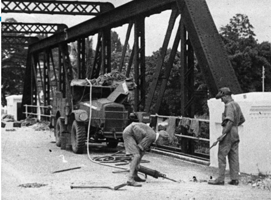
In preparation for the coming Japanese onslaught, British sappers lay explosive charges to destroy a bridge at Seremban along a probable route of enemy advance near Kuala Lumpur in late 1941. BELOW LEFT: British General Sir Arthur Percival (left) was determined to defend Singapore but ultimately surrendered to an invading Japanese army that was inferior in number. BELOW RIGHT: General Tomoyuki Yamashita executed a brilliant advance along the Malay Peninsula and bluffed Percival into surrendering.
