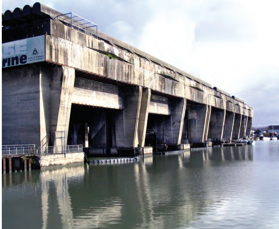
ABOVE: The German U-Boot-Bunker at Bordeaux, France. After the French collapse in 1940, the Regia Marina (Italian Navy) established a top-secret facility here, BETASOM (1940-1943), to improve access to the Atlantic Ocean. Germany, who had the largest submersible fleet in history (1,162 vessels) began building massive reinforced concrete submarine pens here in 1941, making it a major Axis U-boat hub. OPPOSITE: The Regia Marina's Luigi Torelli arrives at the BETASOM sub base in Bordeaux on February 4, 1941, after completing its first Atlantic patrol. She had begun her patrol on November 12, but had to return to base for electric motor repairs after 10 days. She set out again on January 9, 1941.
