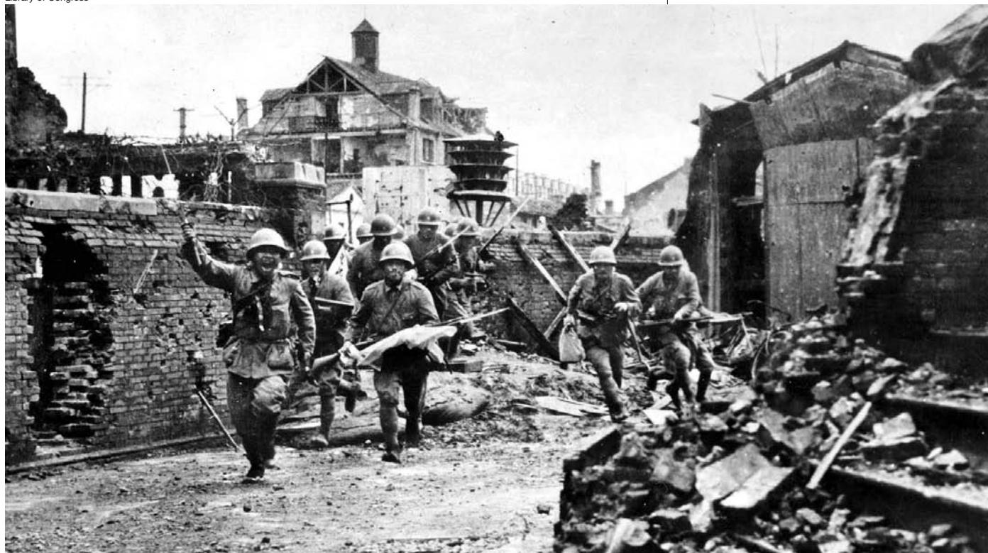
ABOVE: Japanese soldiers rapidly advance through a rubble-strewn street in the city of Toh-an, China. Locked in close combat with Chinese troops, the Japanese pushed toward Kiukang, the terminus of the Nan-Hsun Railway. OPPOSITE: In this Japanese artist's conception of the Battle of Tsushima, sailors of the Imperial Navy fire their weapon at vessels of Czarist Russia's Baltic Fleet. The Japanese victory at Tsushima stunned the world and emboldened the island nation to continue asserting its preeminence in Asia.
