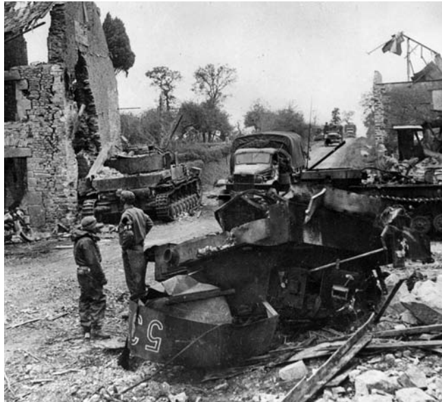
Trucks loaded with fuel for an Allied armored column enter the French town of St. Gilles, rolling past the burned-out hulks of two German armored vehicles. Military Police personnel stand by to direct traffic and keep the supply trucks rolling through the village.
