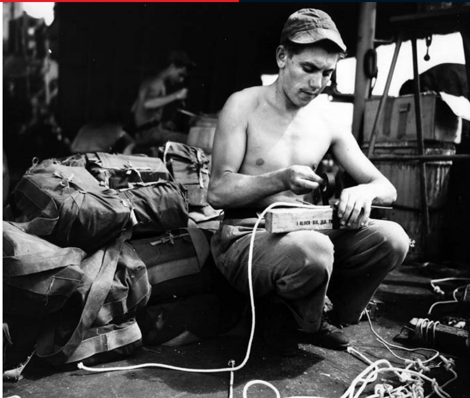
In July 1945, a U.S. Navy UDT team member rigs blocks of explosive TNT for the demolition of beach obstacles at Balikpapan, Borneo. The UDTs operated at Balikpapan in support of amphibious landings by the Australian 7th Division.
