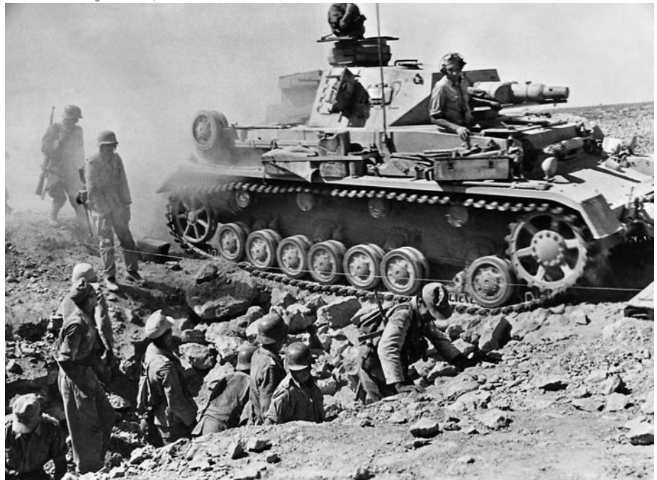
Axis pioneers construct a passage across an Allied antitank ditch during the 1941 Axis offensive against Tobruk.
