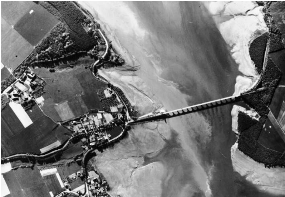
ABOVE: A post-raid RAF reconnaissance photo shows the Mohne reservoir almost completely drained. Hitler authorized the transfer of thousands of workers to clean up the damage and rebuild the dams. TOP: A breach is shown in the Eder Dam on the Weser River in a photograph taken the day following the attack.
