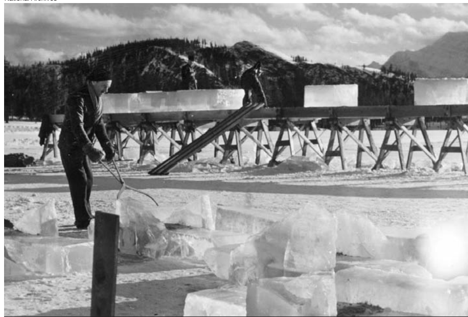
A crew of 15 men spent two months working to build a model aircraft carrier using "pykrete," a mixture of ice and wood pulp, on Lake Patricia, Ontario, Canada in 1943. The construction effort, part of Project Habakkuk, was later abandoned.
